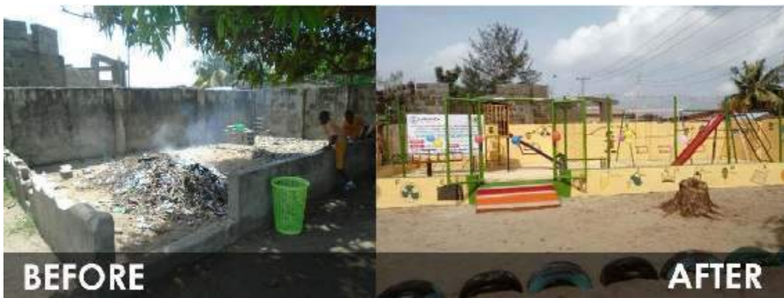
Picture 4: Before and after renovation of Children's Play Court at Community Primary School, Oto-Awori Lagos
